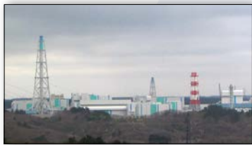
Nuclear reprocessing plant in Rokkasho, Aomori
